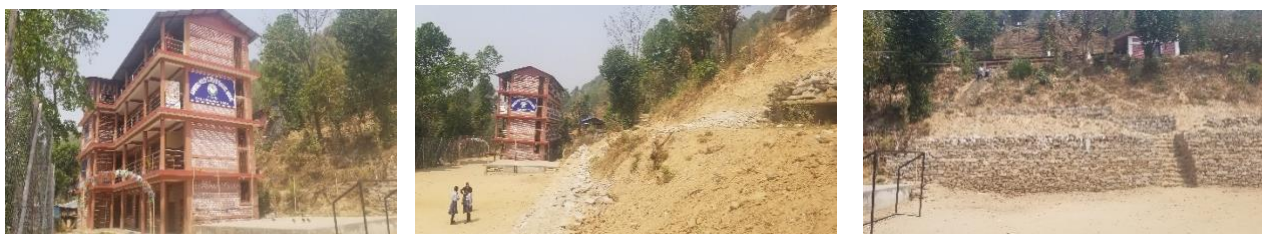
School Building & School Area
