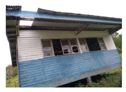
The school building is in very poor condition. The roof is leaking due to extensive damage and missing roofing sheets. Wood in the walls has been damaged by moisture. The lack of a proper fence leaves the building unprotected from cattle wandering in the community. This project will totally replace the metal roofing sheets, install a new chainlink fence
