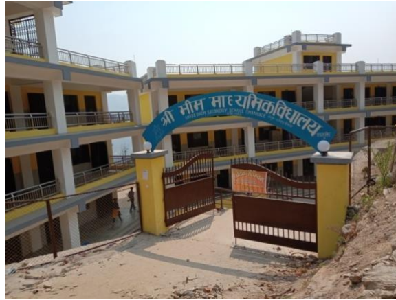
School Area & Buildings
