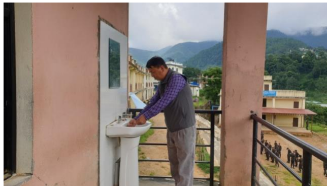
Basin in proper condition
