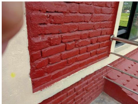
Place where Filtration will be installed
