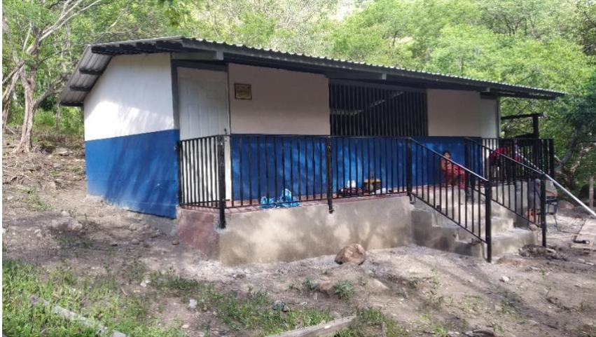
The project will build a 6x10 meter building on the model of the La Pitilla classroom, just finished nearby. See photo at left. It will be made with a concrete foundation, floor and structure, cinder block walls, and metal/zinc roof similar to the photo on the left. Windows will be protected by metal square
