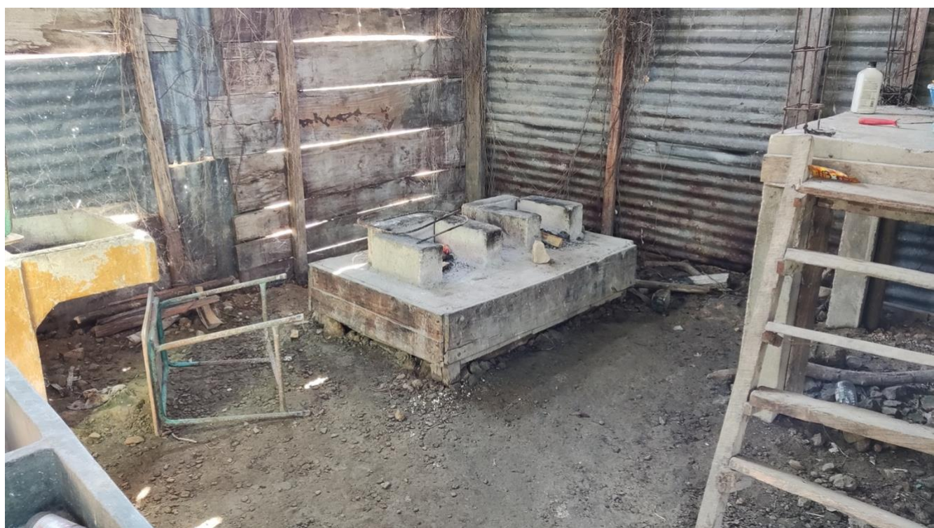
Inside the old kitchen showing the wood burning stove
