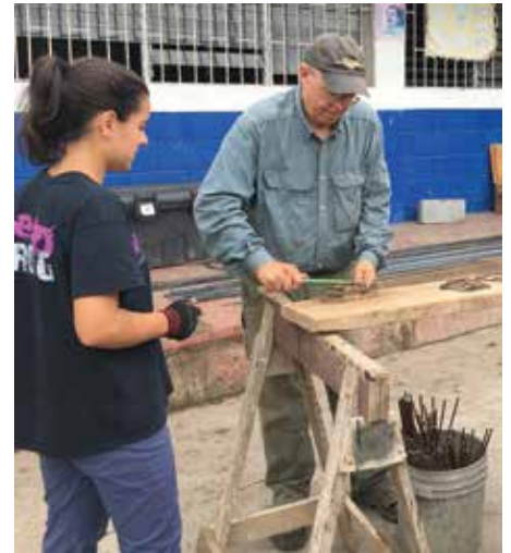
Building a classroom in Nicaragua
