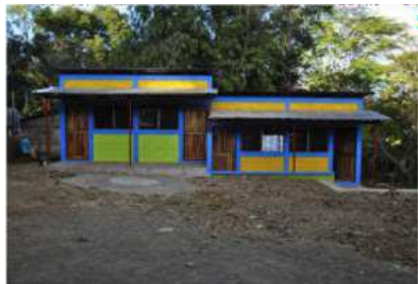
New classrooms Guadalupe Arriba
