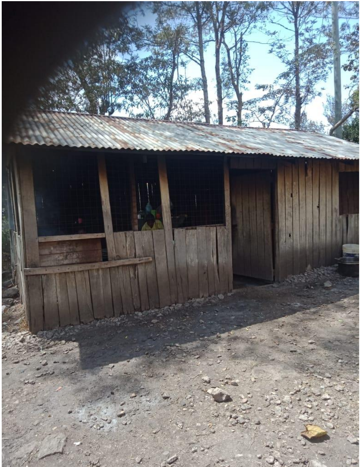
SCHOOL'S MAKESHIFT STRUCTURE THAT SERVES AS THE KITCHEN.
