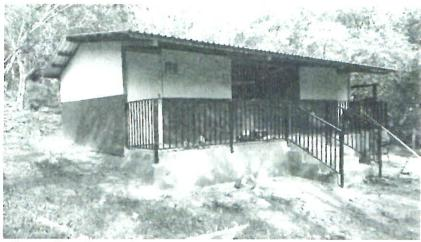
The project will build a 6x10 meter building on the model of the La Pitilla classroom, just finished nearby. See photo at left. It will be made with a concrete foundation, floor and structure, cinder block walls, and metal/zinc roof similar to the photo on the left. Windows will be protected by metal square pipes and doors will be made
