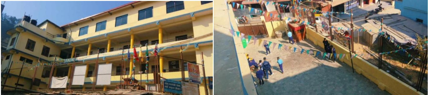
School Building & Compound
