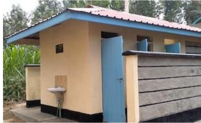
Shining Star Latrines After
