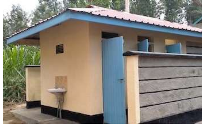
Shining Star Latrines After
